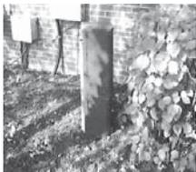
There are areas within the Village where these transformers are blocked by new sod, fences, and even wood piles, which could cause flooding of the unit and possibly a power outage for you and neighbors. If there is an
