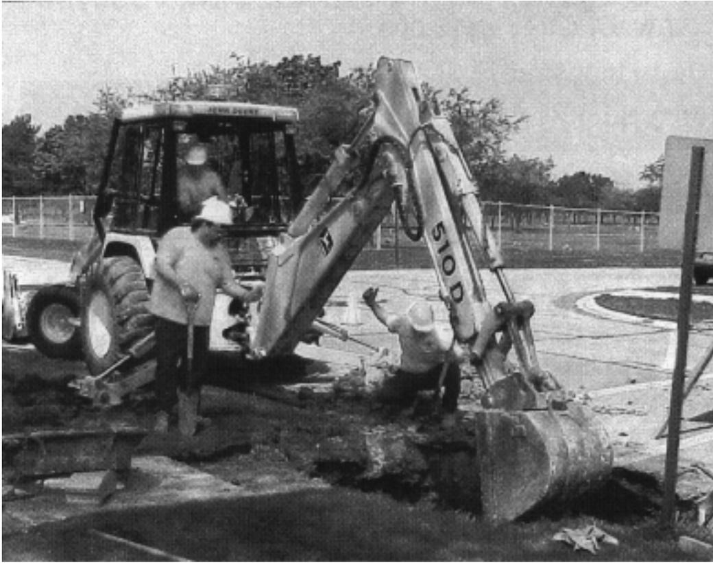
*The Public Works Water Section is always busy maintaining the water system, and making improvements and repairs when needed. Shown here (left to right) are Dennis O'Donovan, Rich Goszczynski and Tom Polcyn installing a water valve basin. Last year, crews repaired 125 water leaks and upgraded 37 fire hydrants along with other projects, such as water valve exercising and installation and other seasonal duties, like snow plowing, branch removal and leaf pick-up.*
