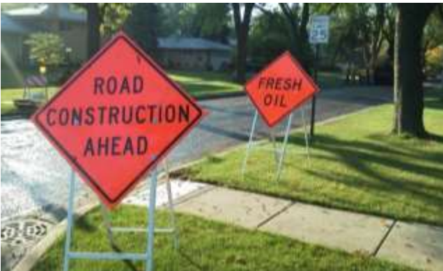
Pay attention to traffic control devices and drive slow.
