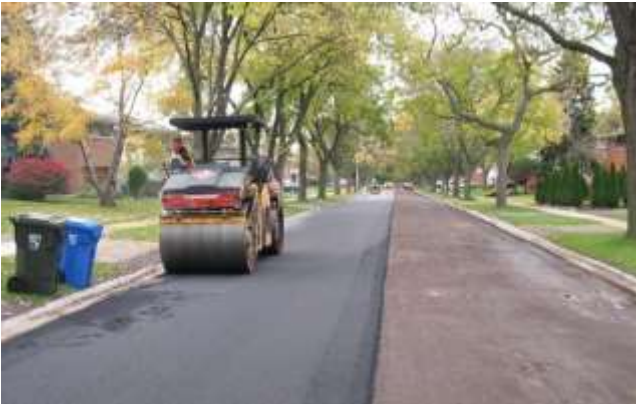
Vibratory roller compacting the first layer of asphalt.
