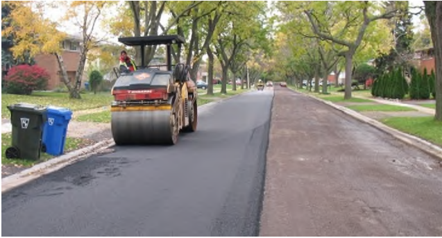
Vibratory roller compacting the first asphalt layer.
