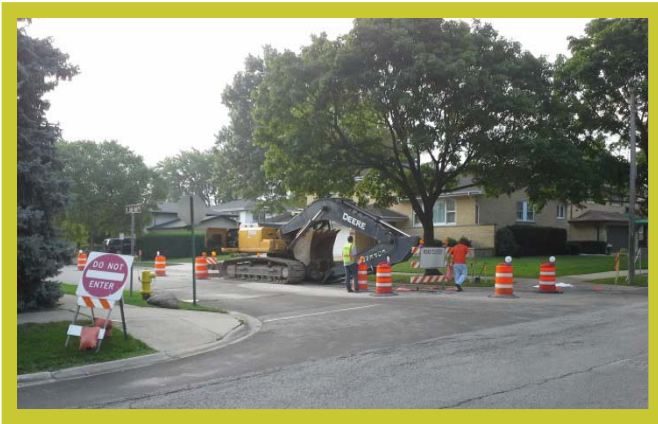
A construction crew mobilizes equipment and traffic control.
